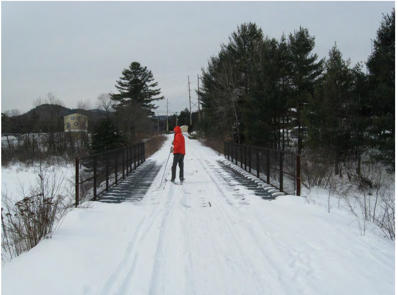
Typical Corridor bridge, 17' between fences, 20' tip to tip across timbers, with open metal grate. Located just west of Lake Placid station
