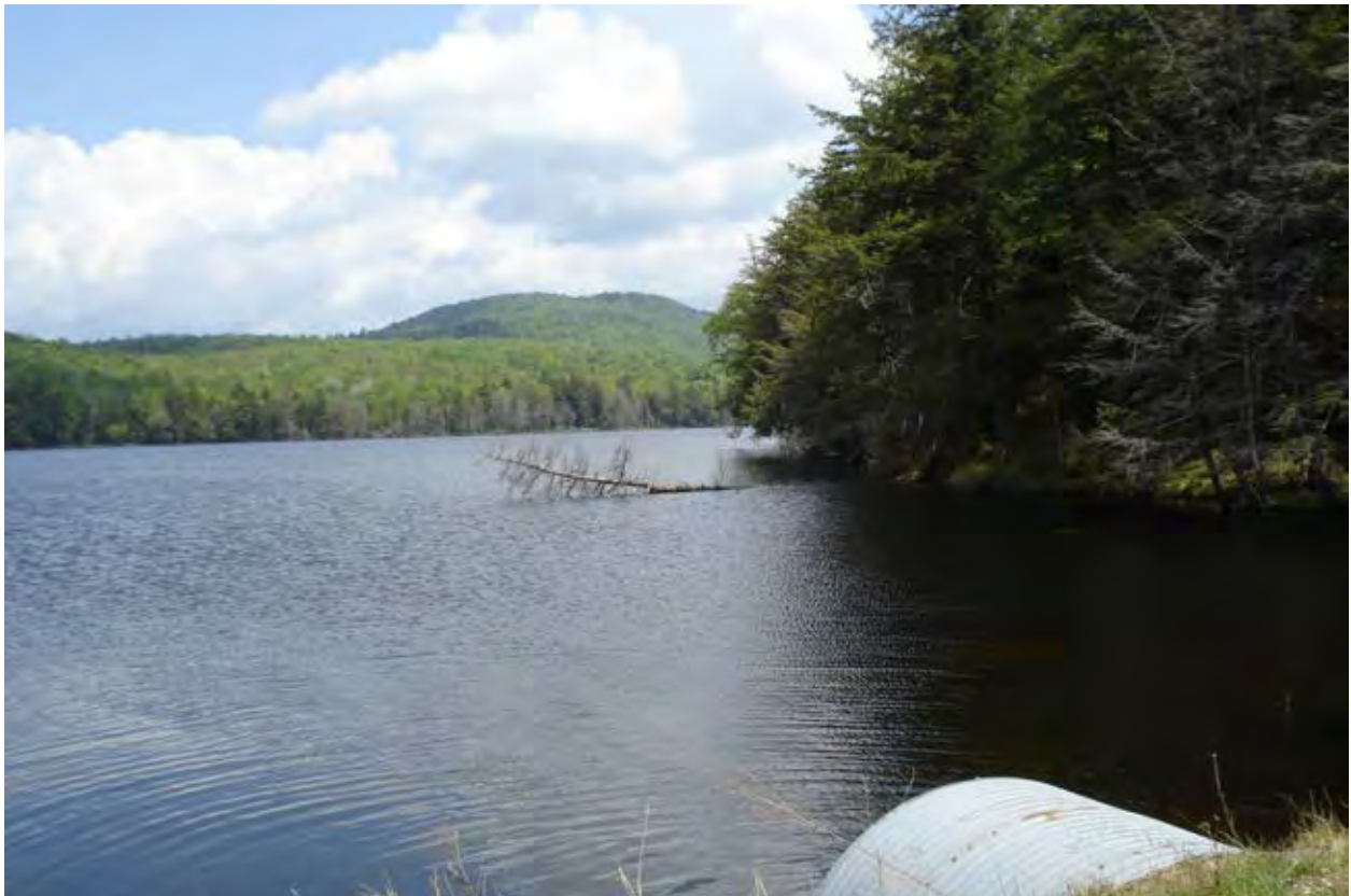
Photo 6: The “Tube” is the culvert between Fourth and Fifth Lakes. Taken from the woods road over the culvert, looking east at Fifth Lake.
