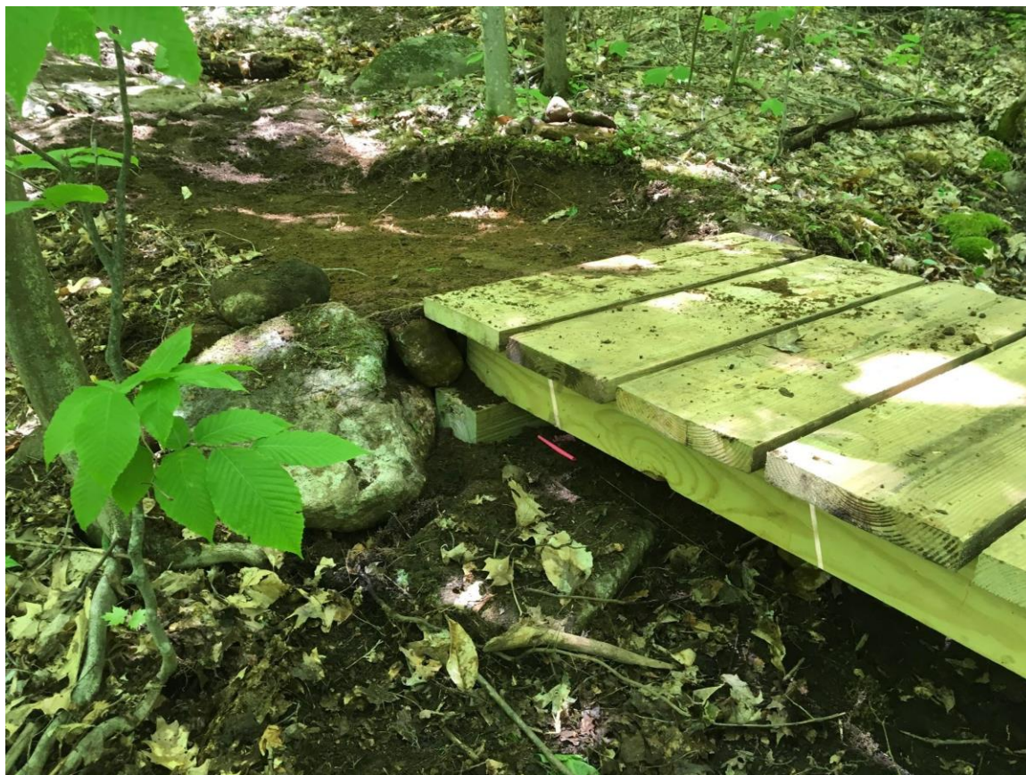
Photo B - Close-up view of the same bridge, showing the transition between the tread and the bridge surface and placement of the bridge sills below grade.
