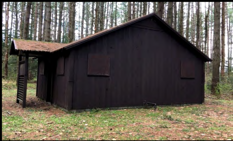
Comfort Station (In Camping Loop)
