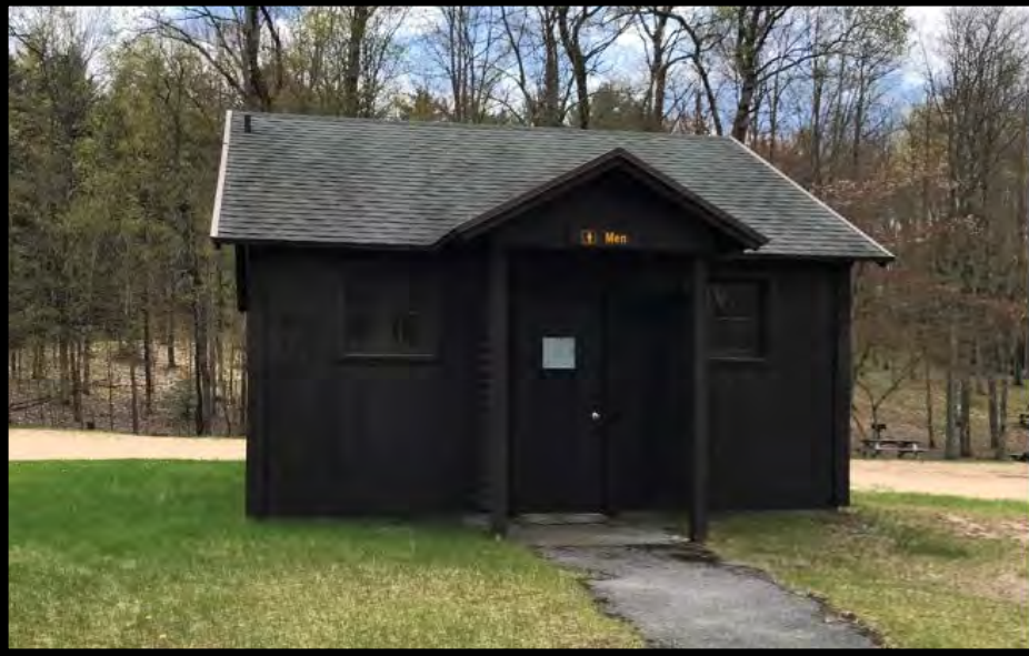
Comfort Station (South of Bathhouse)
