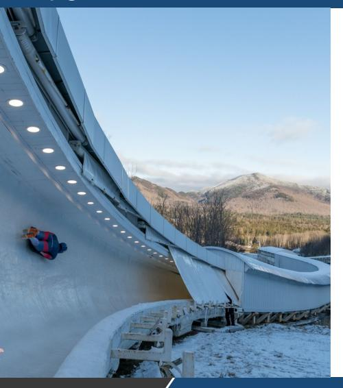
Modern roof and shade systems feature integrated lighting, water, refrigeration and technology
