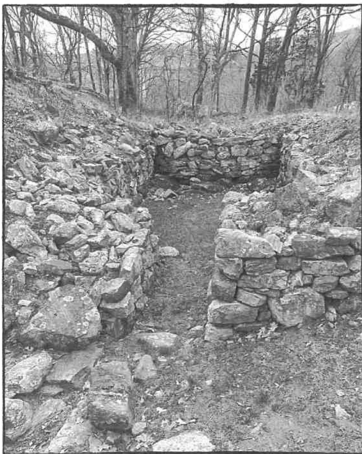
Figure 16. The powder magazine at Fort Montgomery, a revolutionary war feature. These semi-subterranean structures often featured an arched roof that included brick, soil, and sod or soil to protect the powder from incendiary devices (Fisher 2004:115-120).
